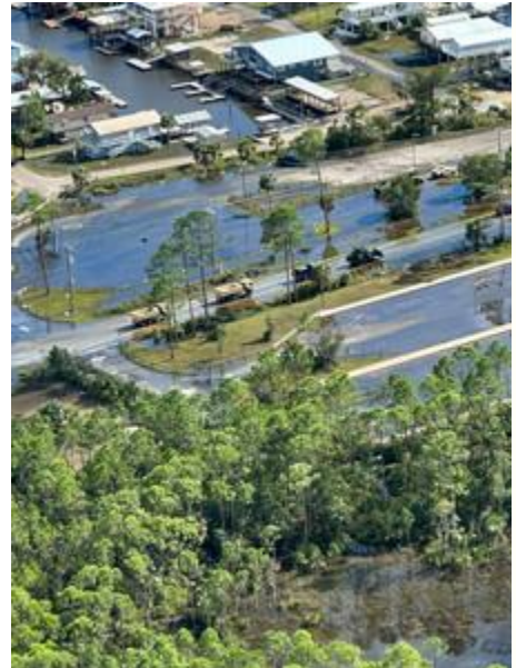
Flooding from Hurricane Idalia in Keaton Beach, Florida. The storm resulted in flooding and damage throughout the communities of Florida's Gulf Coast. [SSG Cassandra Vieira, FLANG, photo]
